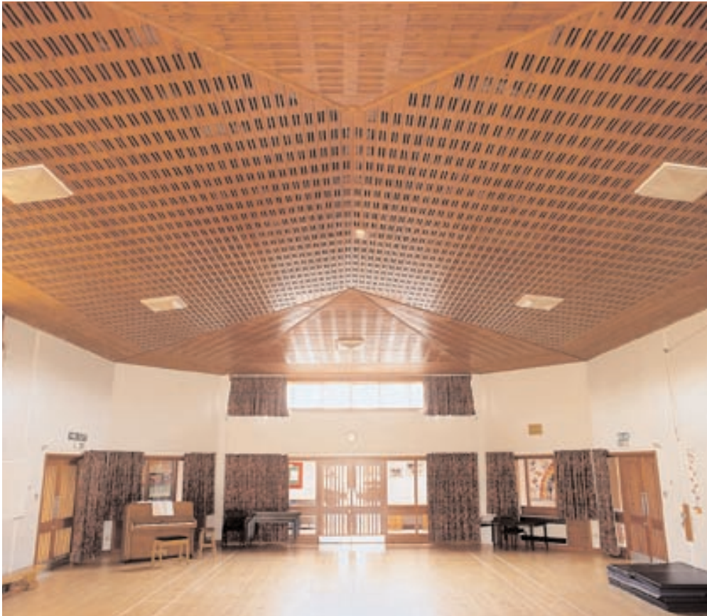
Figure 7.1.3: The hall ceiling after acoustic treatment
