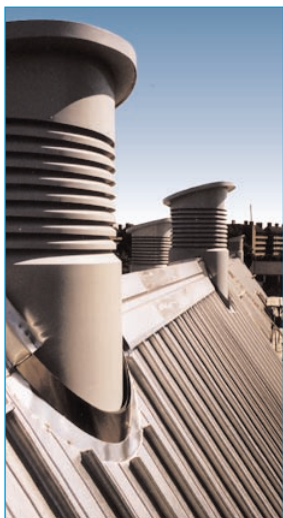
Figure 7.9.4: Three of the roof terminals, during construction
